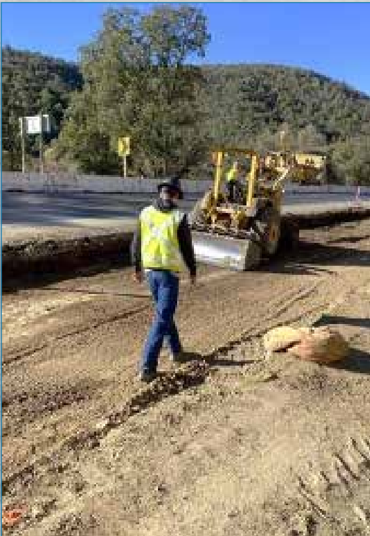
Tribal Member/Monitor David Richter conducting ground survey behind box grader.
