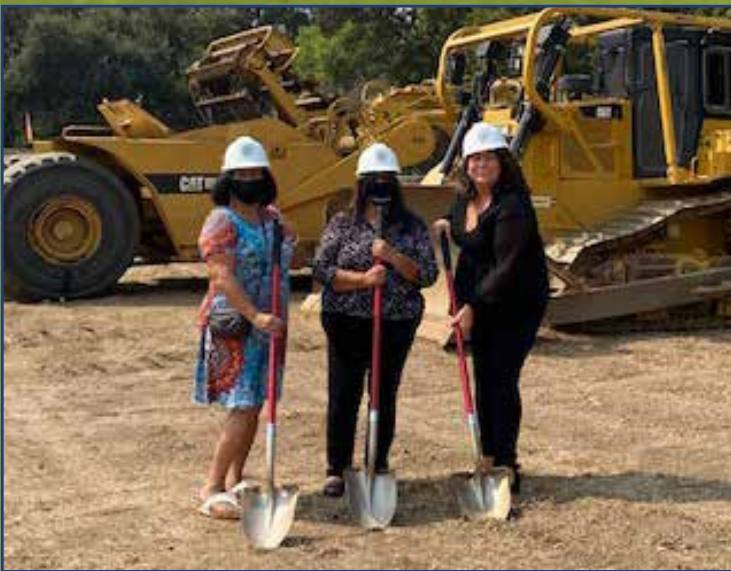
Lake County Tribal Health Consortium Board members and administrative staff were joined by Clearlake City Manager Alan Flora, architects and construction staff for the groundbreaking of the new Southshore Clinic at 14440 Olympic Drive in Clearlake, California, on Tuesday, September 8, 2020.
