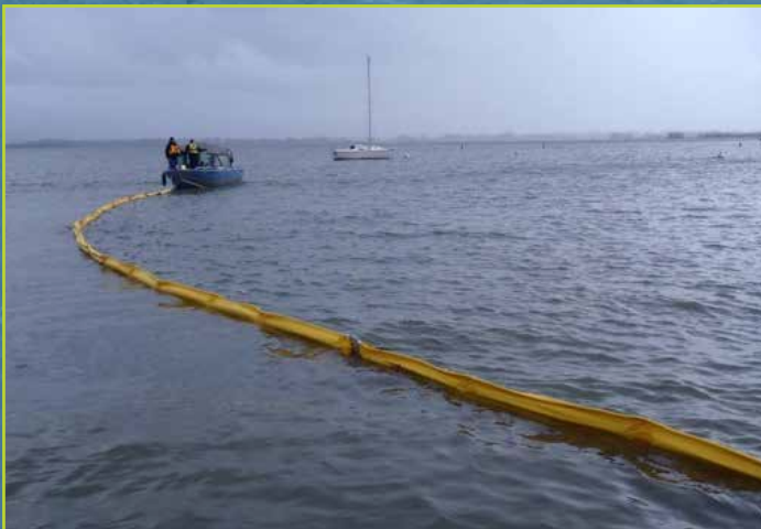
Learning the containment and exclusion technique. Necessary when you are trying to keep surface oil spill in one spot or likewise trying to keep it away from a sensitive area.
